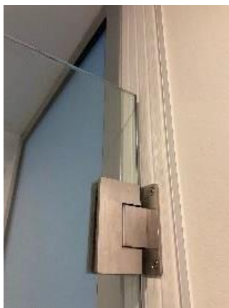
Figure 8: Example of hinges used to support glass door panels and allow them to swing in or out of glass shower enclosures.
