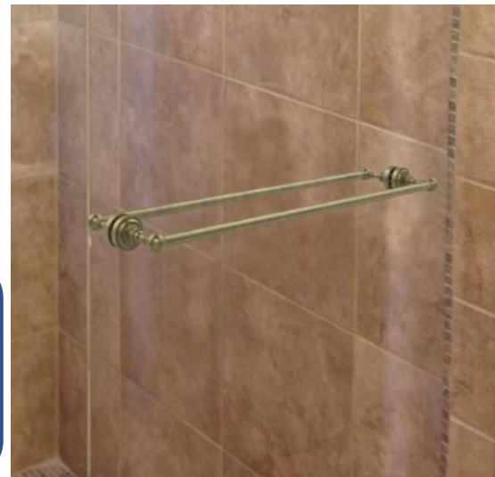
Figure 4: Examples of hardware (handle and horizontal towel bar) on a frameless shower enclosure attached with holes through the glass.
