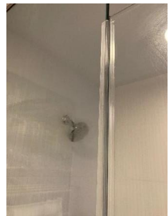
Figure 10: Examples of optional seals (gaskets) used in frameless shower enclosures.
